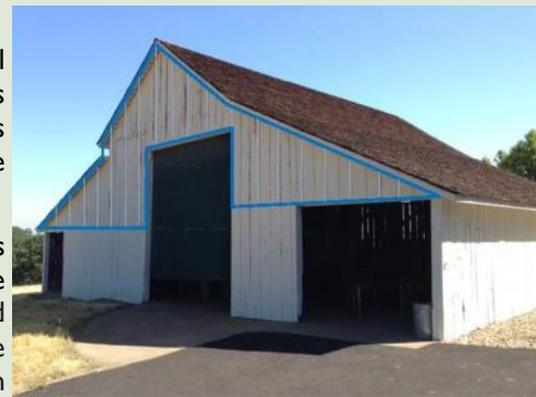
*The blue outline represents the shape of the bird net, after it has been attached and trimmed to size. The net material will be translucent white (not blue) and will stand off approximately 12" from the siding*
